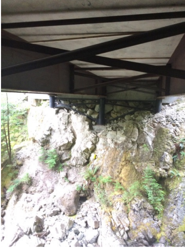
Right Bank Abutment when facing downstream
