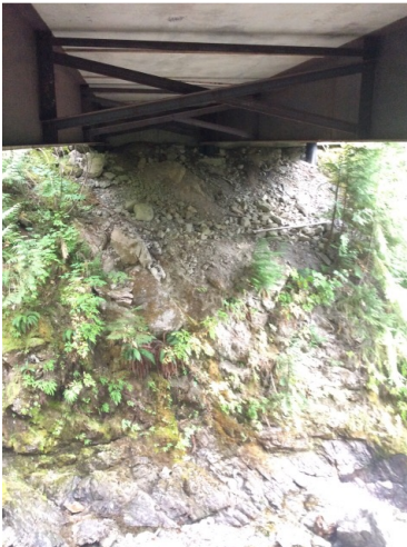
Left Bank Abutment when facing downstream
